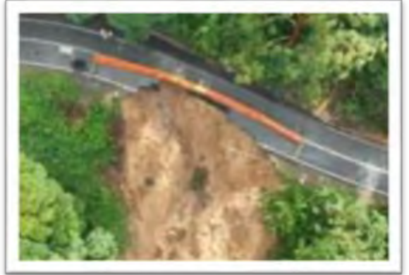
Transport corridors, bridges and embankments
