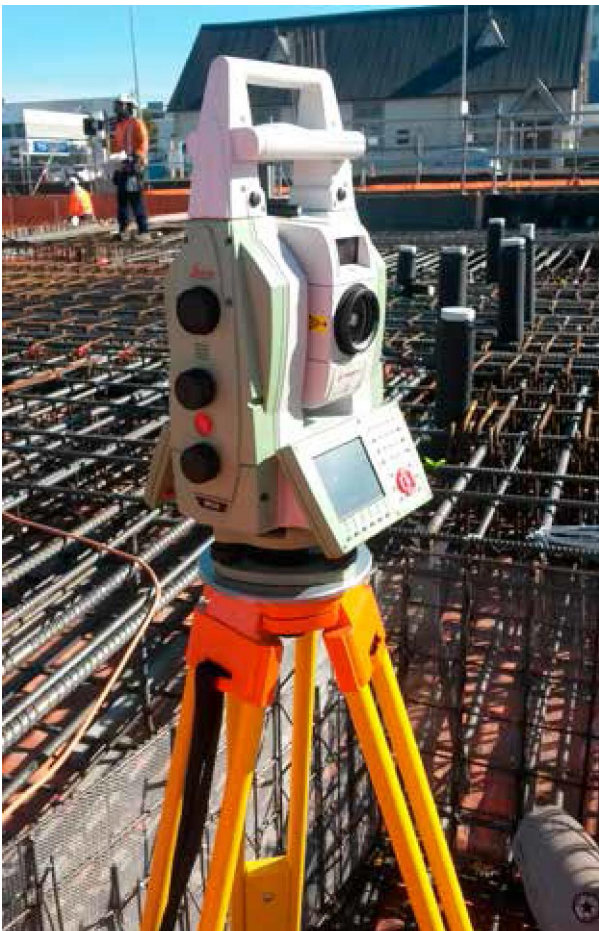
Construction layout and scanner
